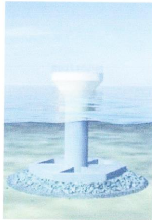
On-gravity-based structure without ballast
